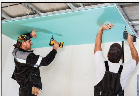
FALSE CEILING & LIGHT PARTITIONS INSTALLATION
