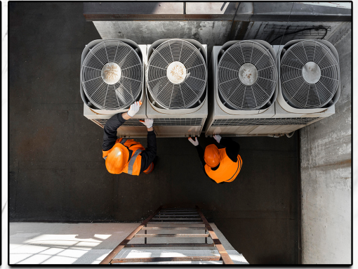
VENTILATIONS & AIR FILTRATION SYSTEMS INSTALLATION
