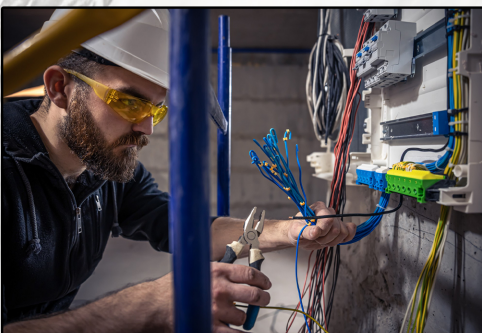
ELECTRO MECHANICAL EQP. INSTALATTION & MAINTENANCE
